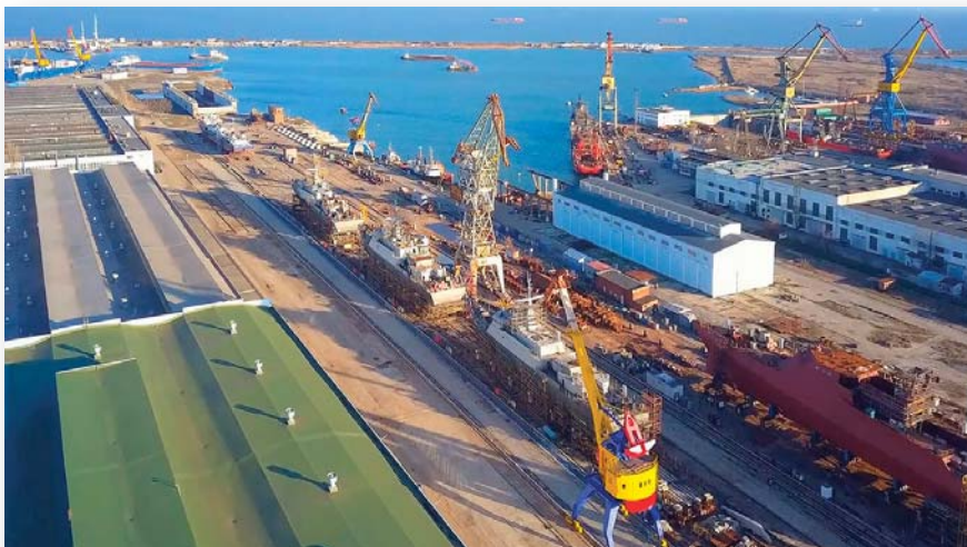
The view of the facilities of the Zaliv Shipyard, februarie 2020, din arhiva BlackSeaNews, https://www.blackseanews.net/en/read/181955
