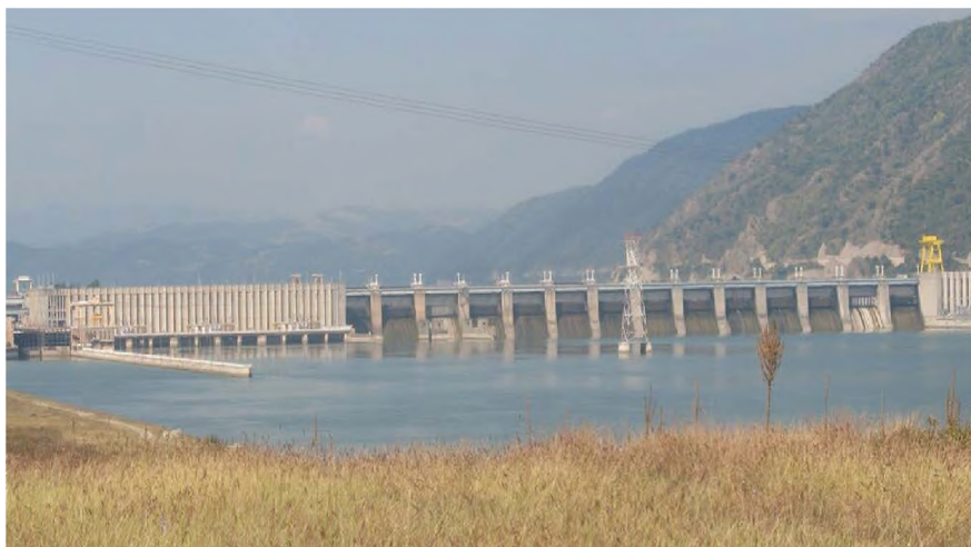
Barajul de la Porțile de Fier I, vedere dinspre Kladovo, https://en.wikipedia.org/wiki/Iron_Gate_I_Hydroelectric_Power_Station#/media/File:HE_%C4%90erdapI_Karata%C5%A1.jpg
